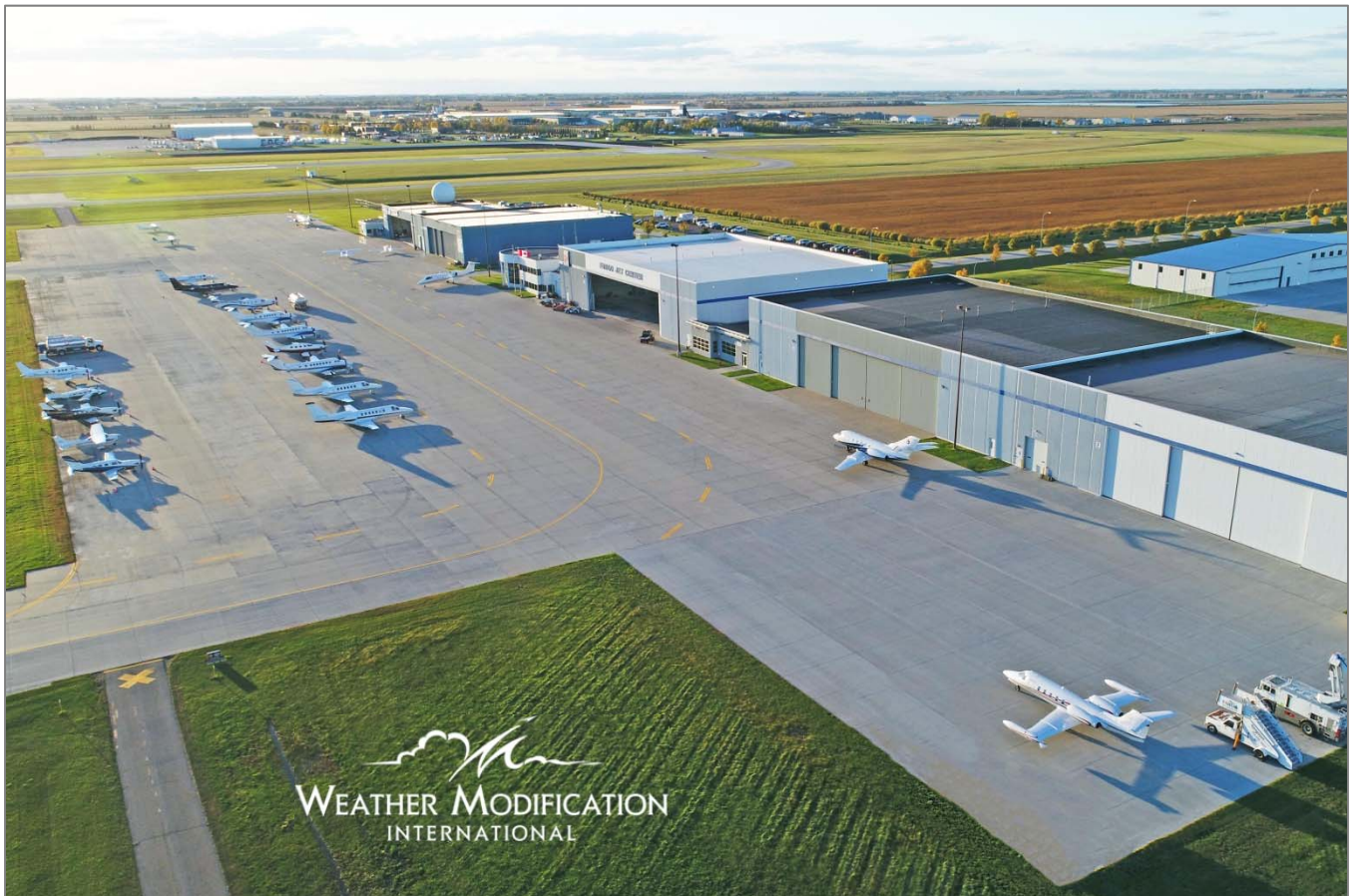
Weather Modification and Fargo Jet Center headquarters on Hector International Airport, Fargo, ND
